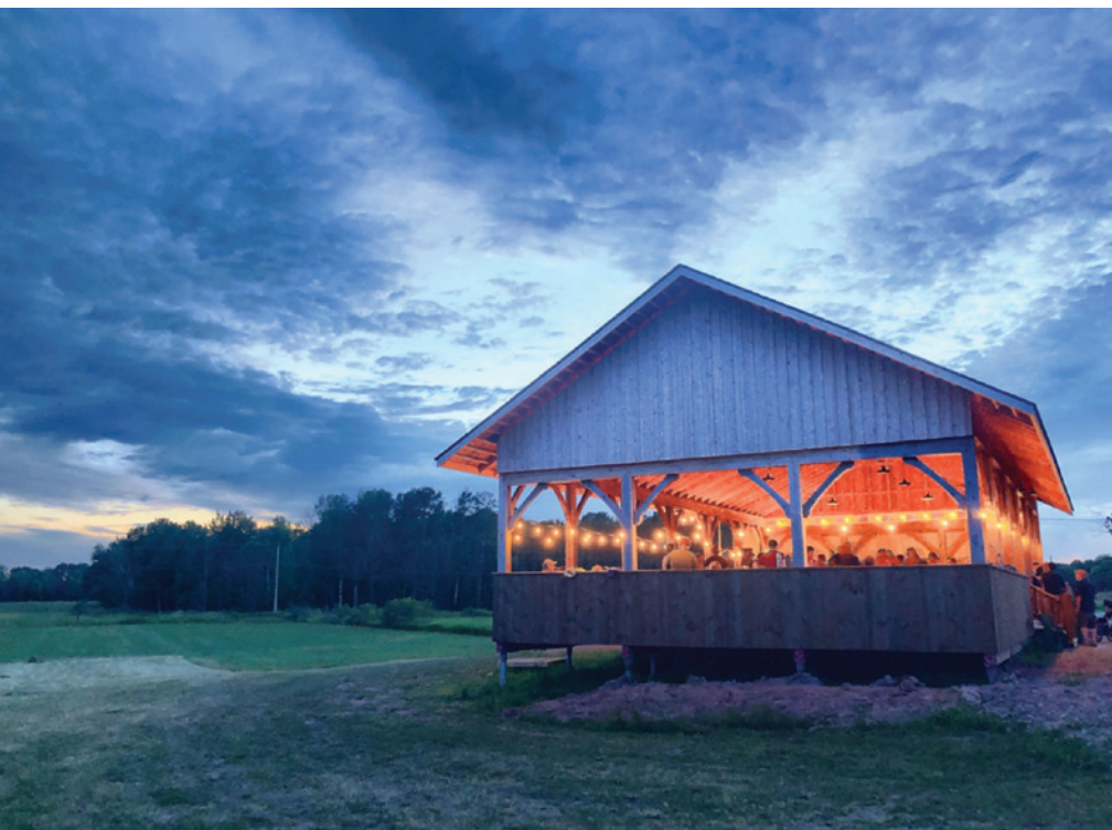
Left: New timber frame dance pavilion built on the 50-Acre site of the future AlgomaTrad Centre, St. Joseph Island. Photos by Vince Candelino.
